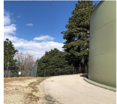
Brookside Wells Figure 4 - SCADA & Data
