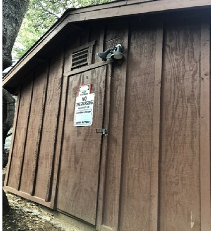
Wabern Pump House - Transfer Only
