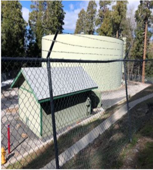
Figure 1 - Chamois Tank Site
