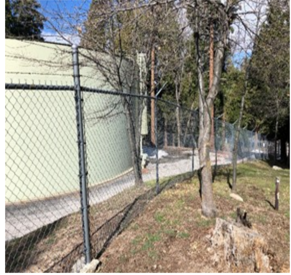
Figure 2 - Chamois Tank and SCADA
