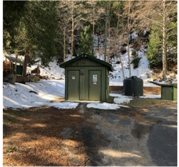
Figure 2 - vertical well and chlorine station
