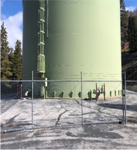
Figure 1 - 2 tanks SCADA and Data Collector
