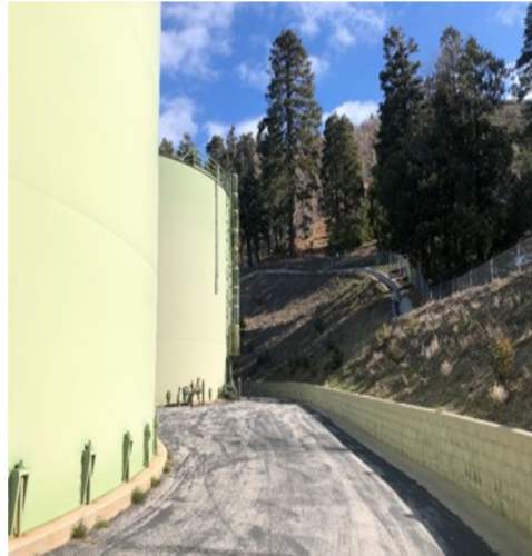
Figure 2 -2 tanks and Data Collector
