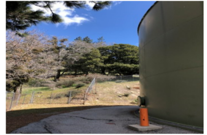
Brookside Wells Figure 1 - SCADA & Data Collection
