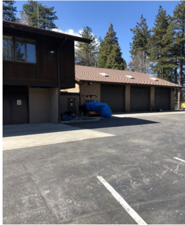
HQ - Rear of OPS Center Figure 1
