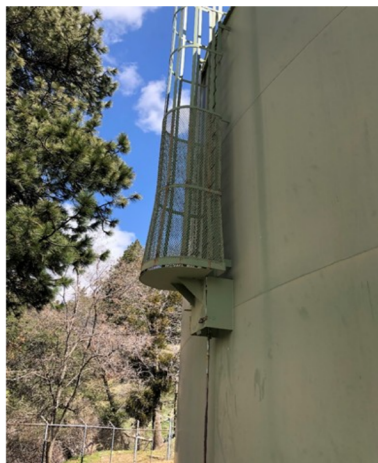
Brookside Wells Figure 5 - SCADA & Data Collection
